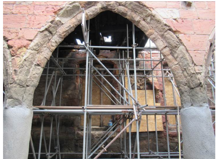
North aisle scaffold- ongoing
