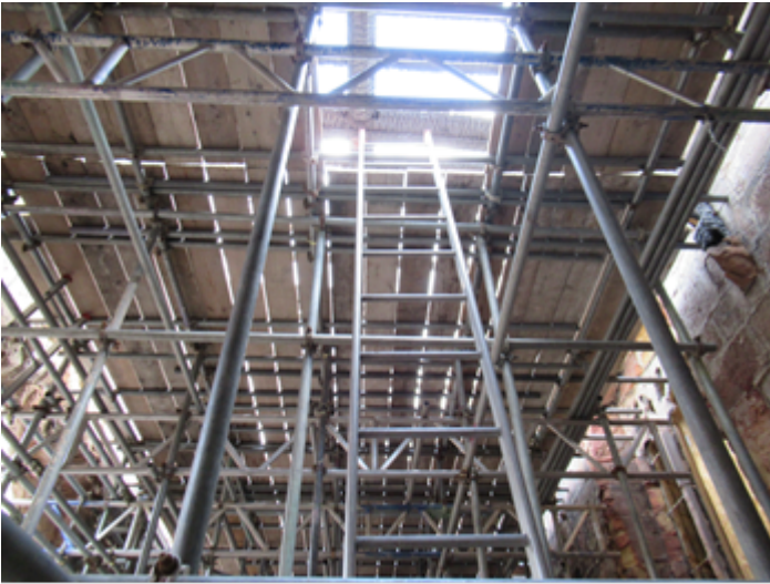
South aisle scaffold
