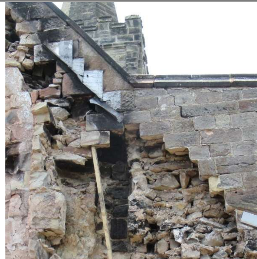
Close up on high-level stone with flue behind
