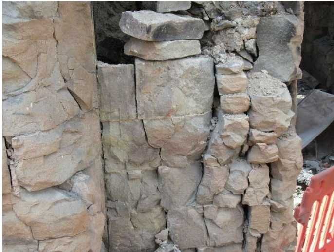
Low level stonework
